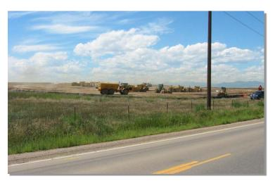
**Photograph VB-1.** A vegetated buffer is maintained between the area of active construction and the drainage swale. Photo courtesy of WWE.
